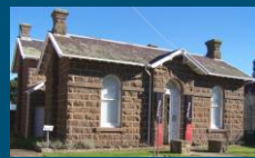
Penhurst Volcanoes Discovery Centre in historic "bluestone" former Offices of Share of Mount Rosier (1864). (Photograph: © Mac Web Service 2012)
