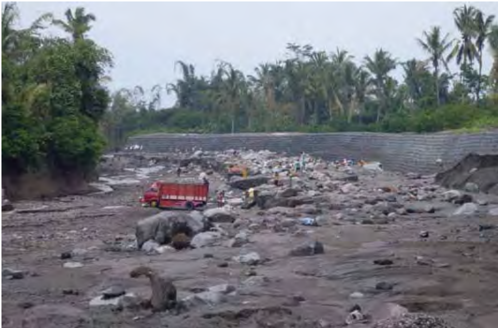
Figure 26: Strengthening of river embankment in Indonesia using volcanic materials deposited during the 2010 eruption of Merapi. Photo by Vittorio Bosi.
