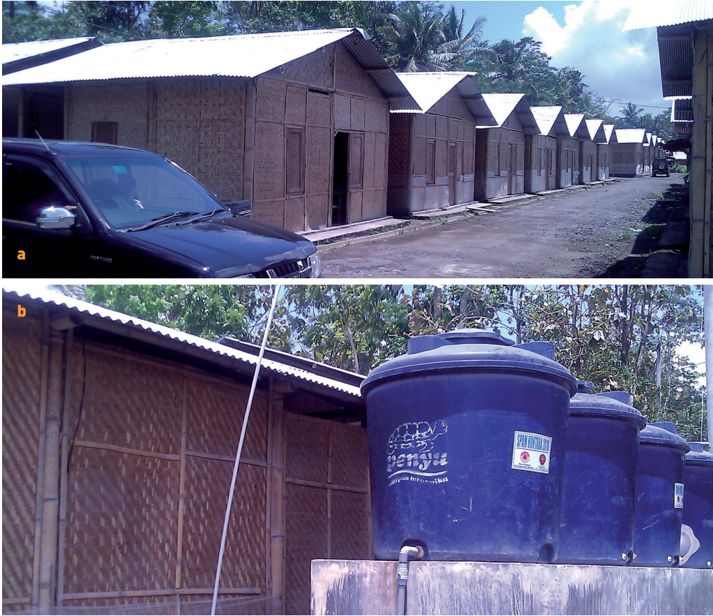
Figure 23: a Provisional houses built in Indonesia after the 2010 eruption of Merapi volcano; b water supply system for the provisional houses. Photo by Vittorio Bosi.
