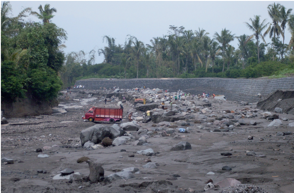
Figure 26: Strengthening of river embankment in Indonesia using volcanic materials deposited during the 2010 eruption of Merapi. Photo by Vittorio Bosi.
