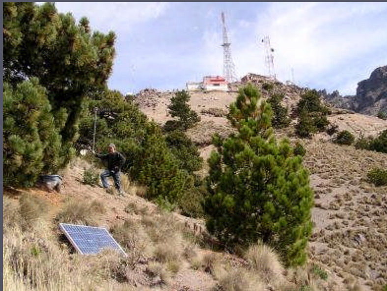
Installing infrasound station
